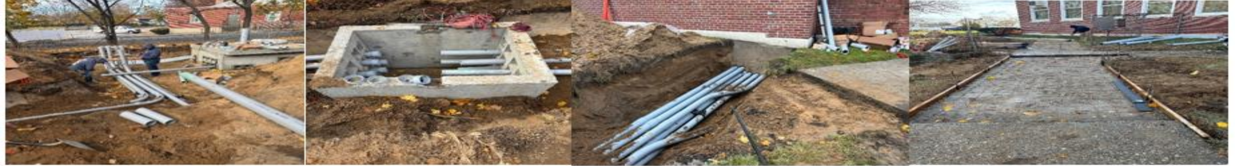
Electrical Underground Piping and Transformer Pad
