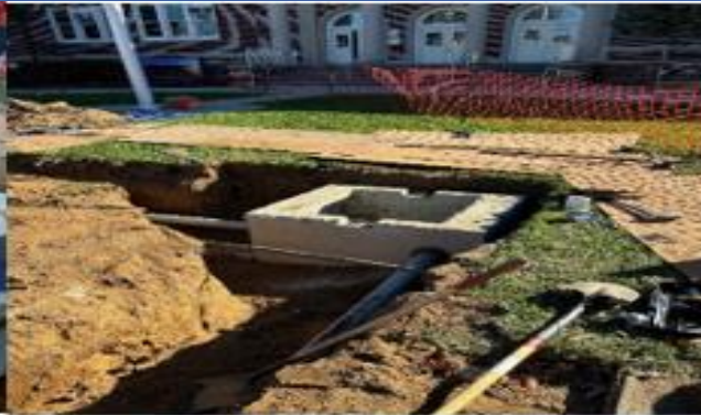
Electrical Underground Piping and Transformer Pad
