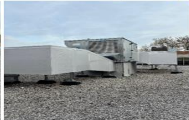
Rooftop HVAC Units, Insulated, and Waterproof Ductwork
