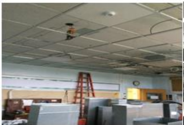
New Suspended Ceiling Grid
