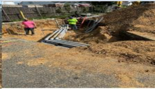
Electrical Underground Piping and Transformer Pad
