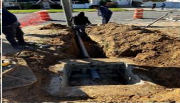
Electrical Underground Piping and Transformer Pad
