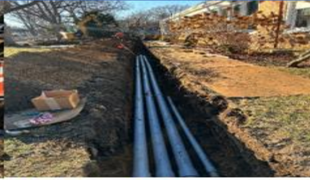
Electrical Underground Piping and Transformer Pad
