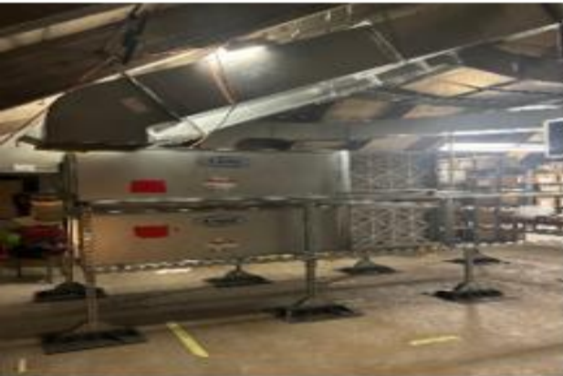
Dedicated Outdoor Air Systems (DOAS) Equipment and Ductwork in Attic Space
