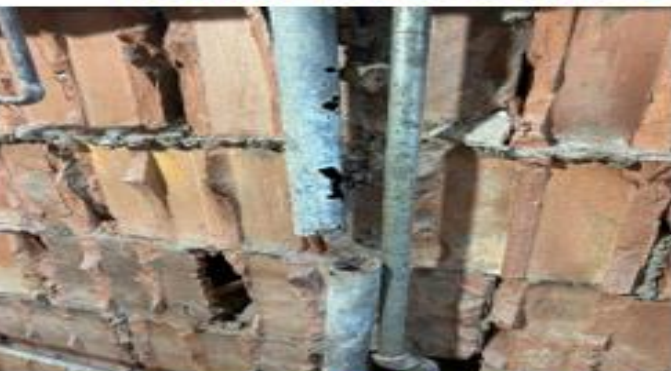
Rotted Piping Found Behind Walls
