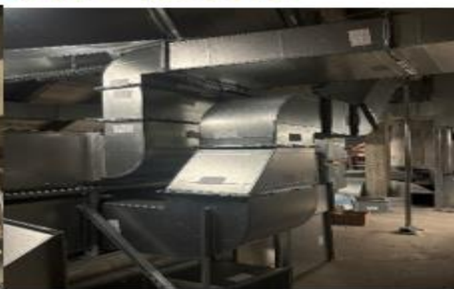
Dedicated Outdoor Air Systems (DOAS) Equipment and Ductwork in Attic Space
