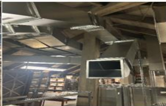
Dedicated Outdoor Air Systems (DOAS) Equipment and Ductwork in Attic Space
