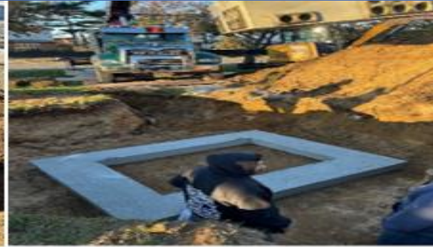
Electrical Underground Piping and Transformer Pad
