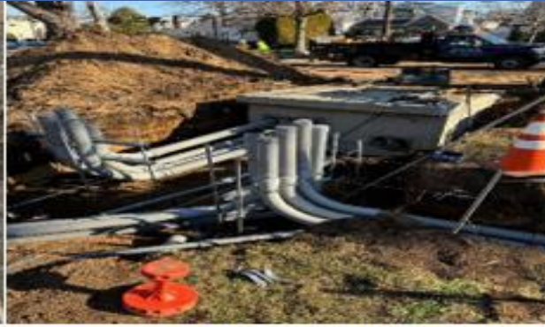
Electrical Underground Piping and Transformer Pad
