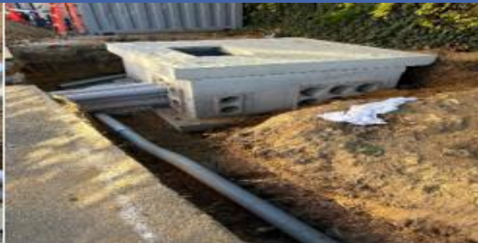
Electrical Underground Piping and Transformer Pad
