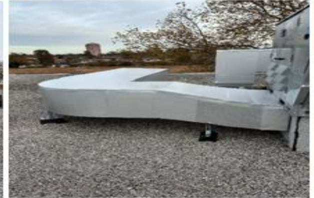
Rooftop HVAC Units, Insulated, and Waterproof Ductwork
