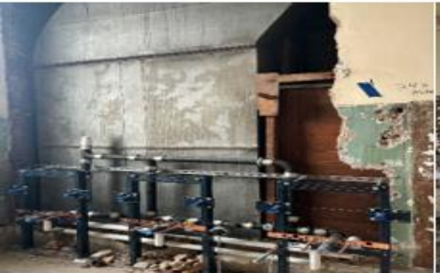
Restroom, Demolition, New Plumbing
