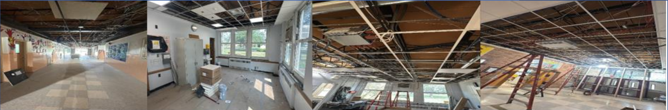
CLASSROOMS, CORRIDORS UNDER CONSTRUCTION
