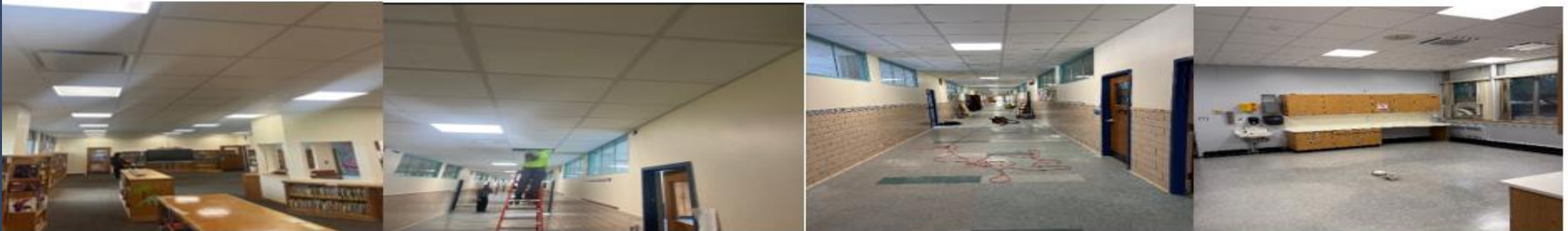
NEW CEILINGS AND LIGHTING IN CORRIDORS, LIBRARY, CLASSROOMS, AND OFFICES
