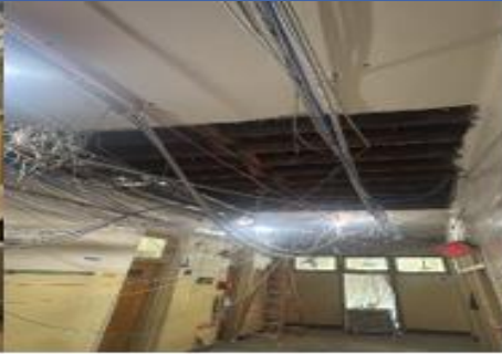
ALL CORRIDOR CEILINGS BEING REPLACED
