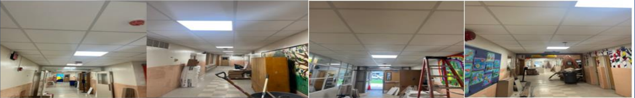
NEW CORRIDOR CEILINGS AND LIGHTING
