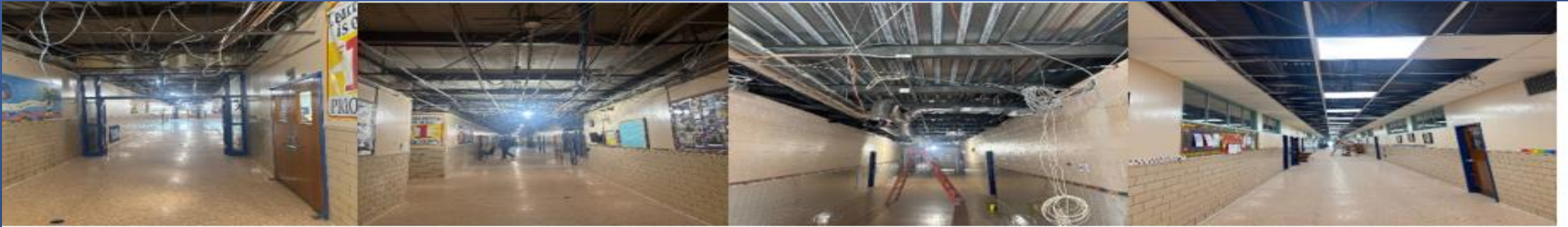
CORRIDOR CEILINGS REMOVED AND REPLACED
