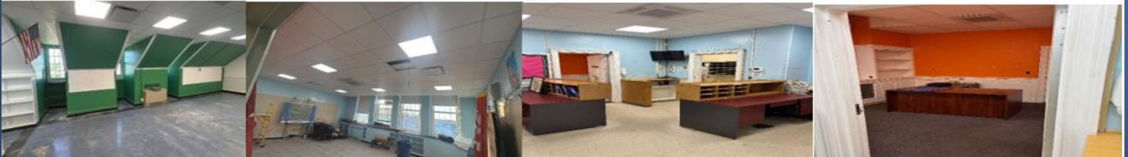
New Classroom Ceilings and Lighting
