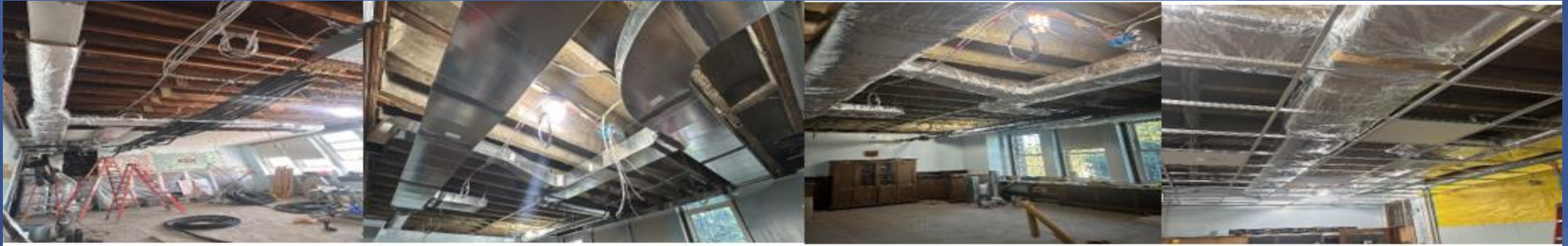
NEW DEDICATED OUTDOOR AIR SYSTEMS DUCTWORK
