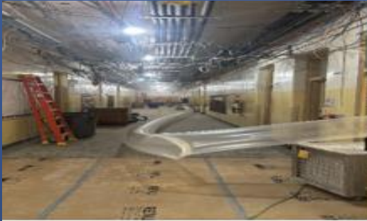
ALL CORRIDOR CEILINGS BEING REPLACED
