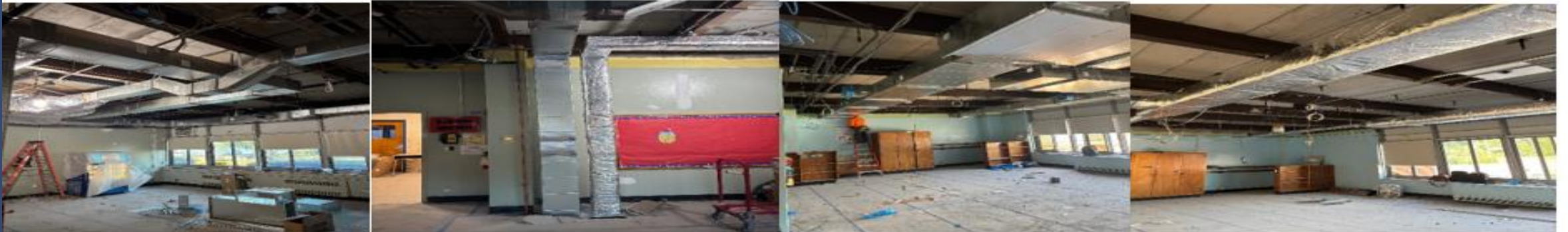
NEW DEDICATED OUTDOOR AIR SYSTEM (DOAS) DUCTWORK
