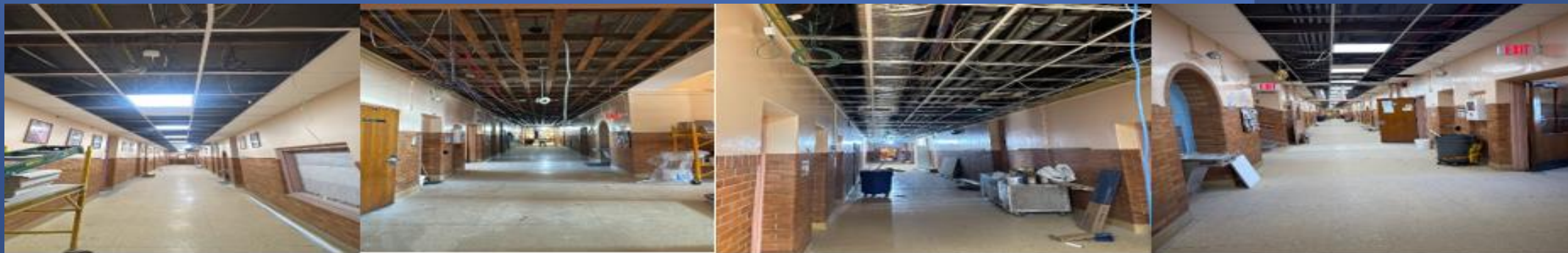
CORRIDOR CEILINGS REMOVED AND REPLACED
