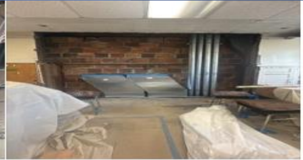
SHAFTS FROM BASEMENT TO ROOF
