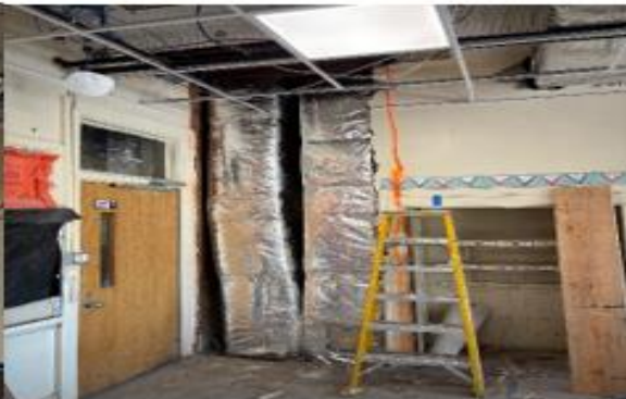
DUCTWORK IN SHAFTS
