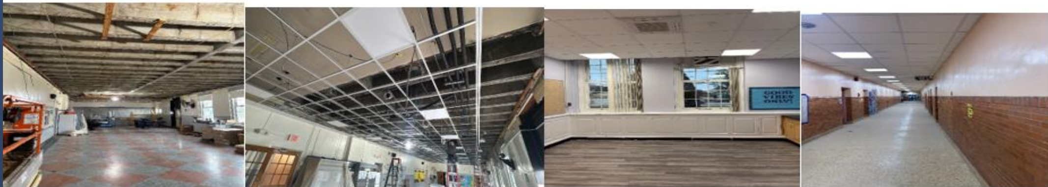
CAFETERIA, NEW CEILINGS, LIGHTING, HVAC
